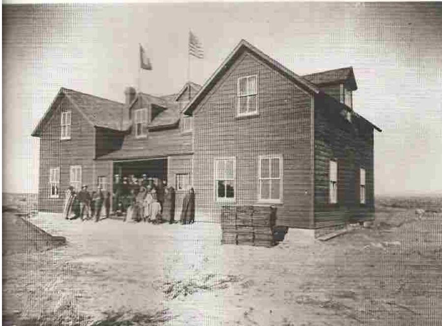
Original mission school building, which burned in 1900 (ISHS)
